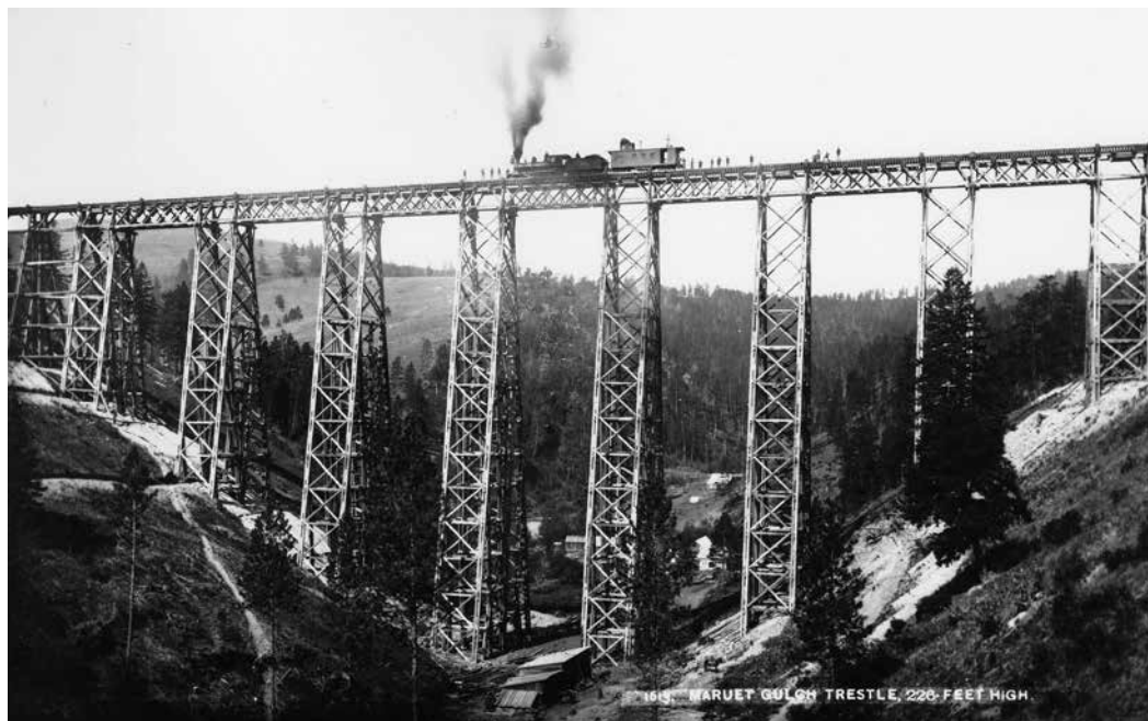
The Northern Pacific Railroad's newly constructed Marent Trestle, near the southern border of the Flathead Indian Reservation, 1884. Francis Haynes photograph, courtesy Montana Historical Society.
