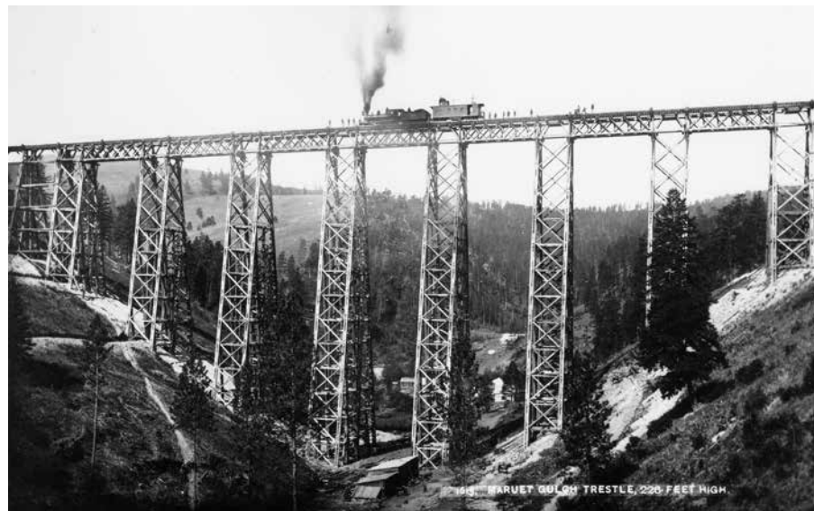
NPRR's Marent Trestle near southern boundary of Flathead Reservation, 1884. Photograph by Francis Haines, courtesy Montana Historical Society Research Center.
