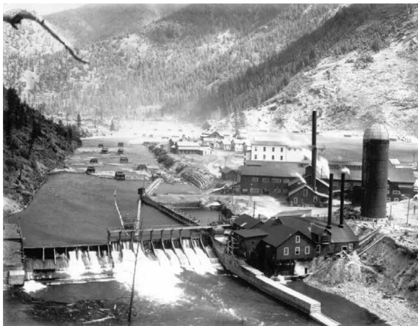
Dam by the Big Blackfoot mill, and log rafts in river, n.d., but before 1908. Photo by Morton J. Elrod, courtesy Archives and Special Collections, Maureen and Mike Mansfield Library, University of Montana - Missoula.
