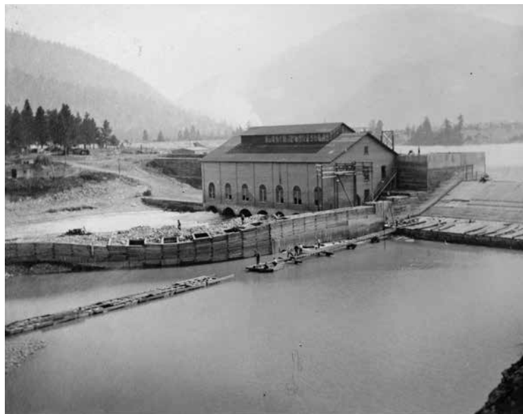
The newly completed Milltown Dam, April 1909. Library of Congress.
